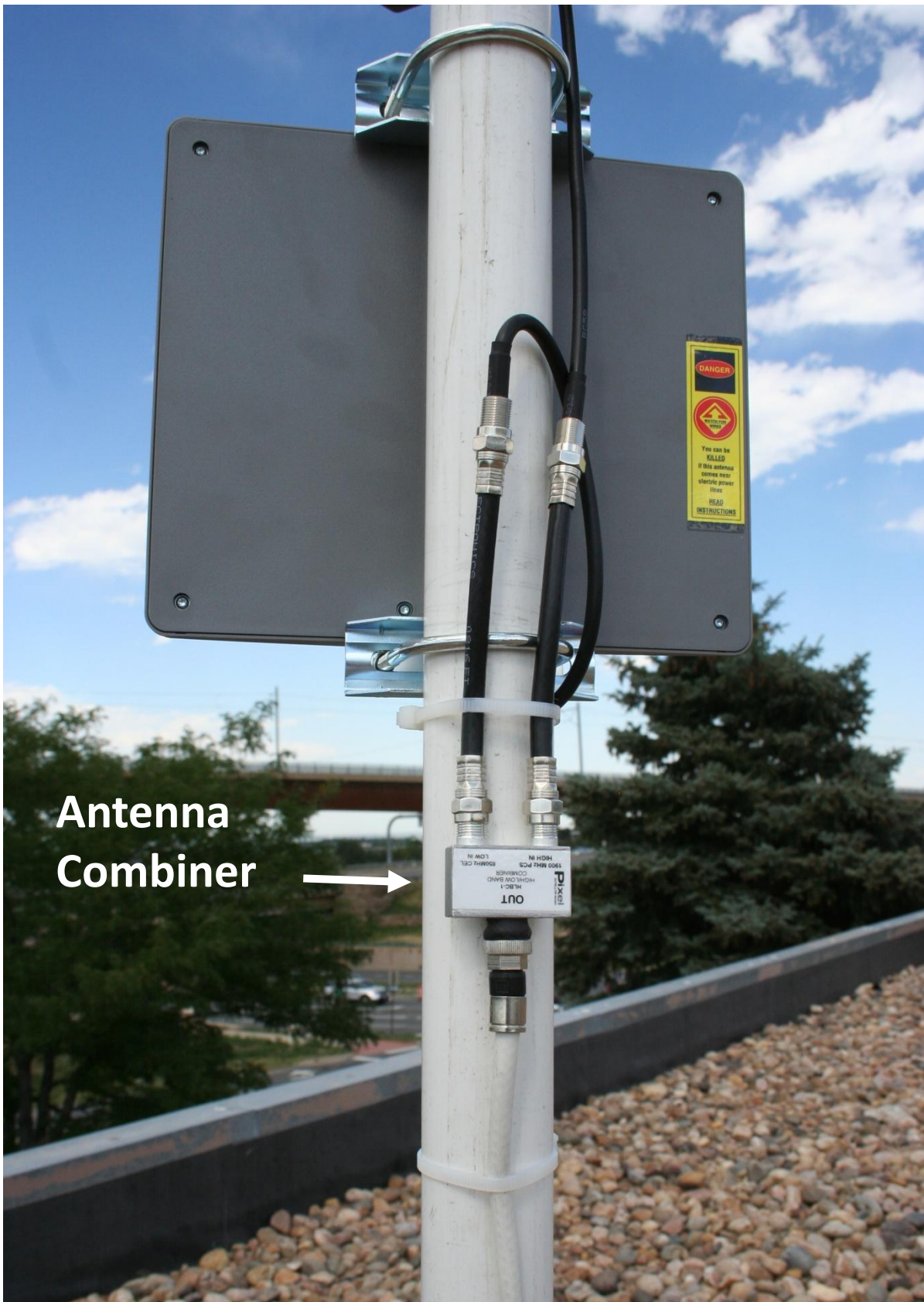
Figure 10. Outdoor Panel Antennas Connected to Diplexer
